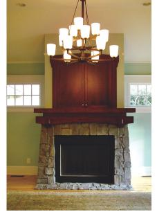
The chimney for the home's existing coalburning fireplace was rebuilt and a gas-fired coal basket insert installed to replace the original. The new surround and hearth features a tumbled marble finish. The fireplace's original mahogany mantle was refinished on-site.
