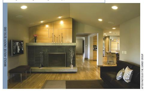
The original fireplace was completely disassembled and rebuilt with a solid pour concrete hearth and mantel, limestone tile face and white oak upper cabinetry panels. "The only part we kept was the firebox," says remodeler Bob Mock.
