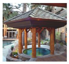
Designing the spa required skilled craftsmanship. Discrete knife joints were used to connect the logs without visible nails.
